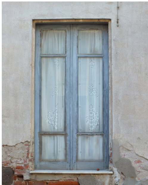
Via Carmine, finestra architravata
