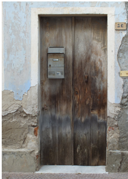
Via Angioy, porta architravata
